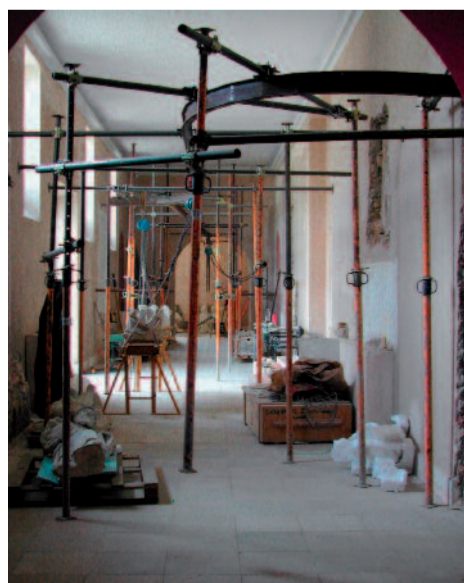
The system used to de-install the altarpieces
