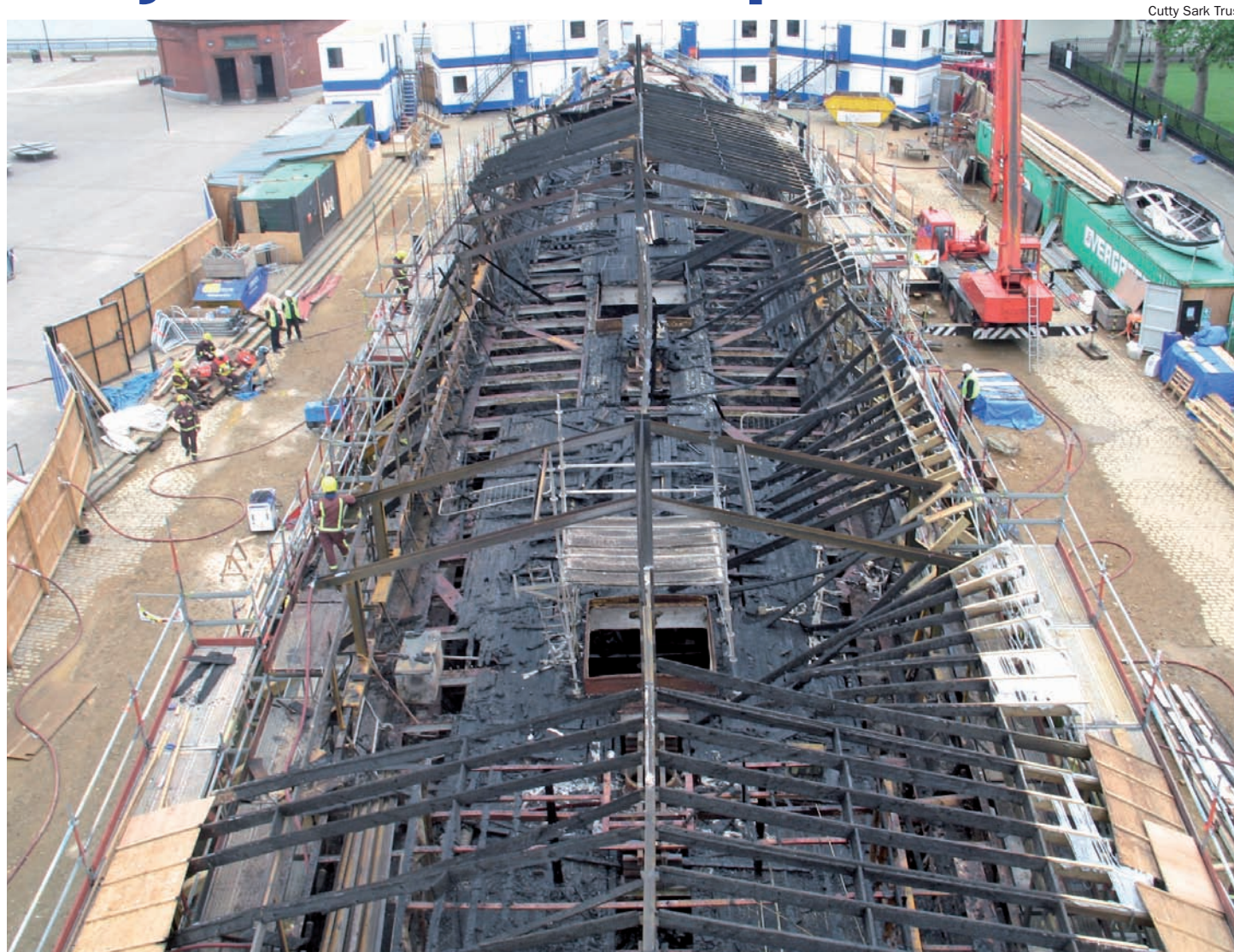
An aerial image of the main deck showing the extent of the fire. It remains to be seen how much damage the ironwork has sustained
