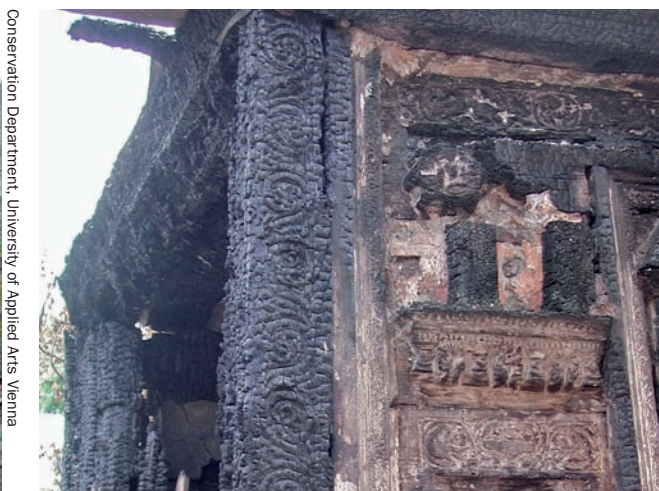
The elaborately carved wooden entrance portal suffered extensive damage in the fire
