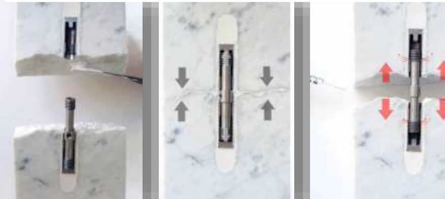
Figures 7, 8 and 9. Application of adhesive/ releasing the pin
