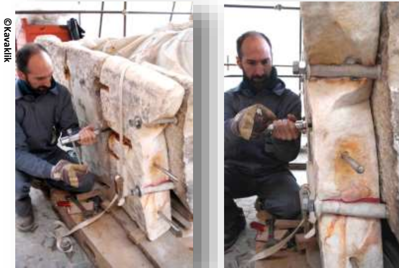
Fig.1 and 1b - Insertion of threaded pins into exterior-opening holes (red arrow) and "dry" (no adhesive) pins (blue arrow). With thanks to the firm Kavaklik (Works direction - Vatican Museums).
