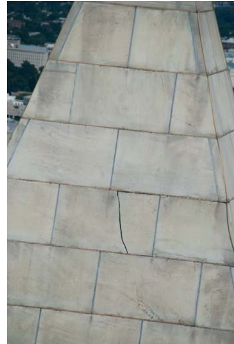
An image taken by a U.S. National Park Service helicopter, showing cracks in the Washington Monument in Washington, D.C., in the United States.
