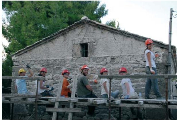
Removing the cement joints
