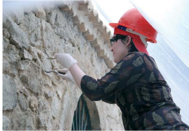
Not even the rain can stop us from saving the stone masonry!
